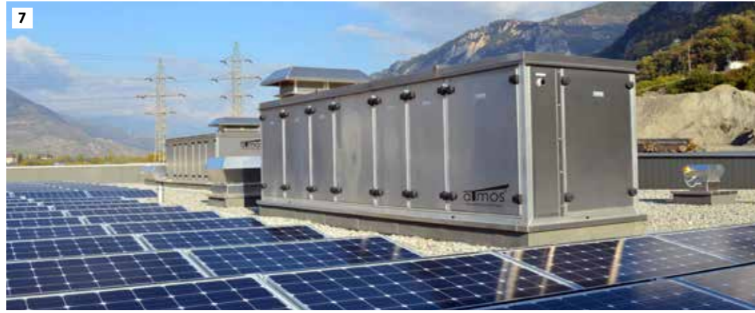
++ Hygienic, biological air ventilation system outside the facility
